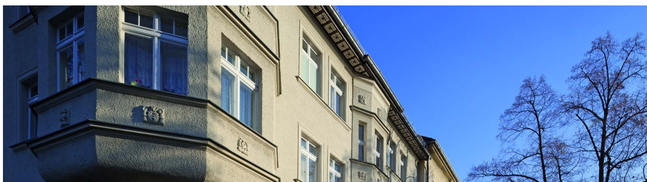
The Germany property company Deutsche Wohnen was the best contributor to SKAGEN m2 last year. Pictured here is one of the company's properties, a hospital complex in Berlin.
